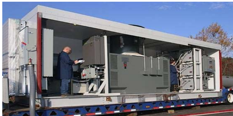
Figure 4: Voltage and transient stability control technology, high temperature superconducting (HTS) synchronous condenser. American Superconductor at TVA. Image is courtesy of TVA and AMSC.
